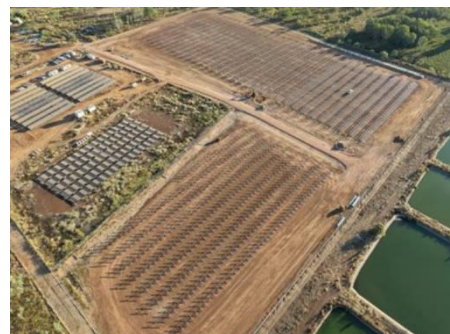
The expansion of the Doomadgee Solar Farm is progressing well, with the civil works completed by the local council and the infrastructure for the solar panels now installed.
