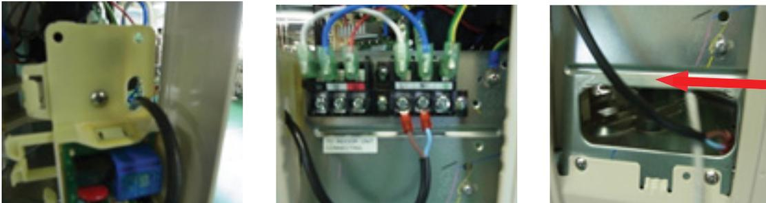
Paste filament tape on the edges to prevent it from cutting the wires
