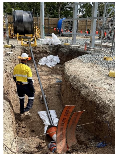
Fig 1 – An example of an underground 66kV cable being pulled through conduit.
