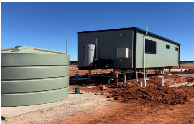
New amenities building at the Boulia Solar Farm.
