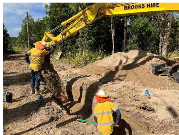
Fig 1 – Contractors installing lengths of conduit.
