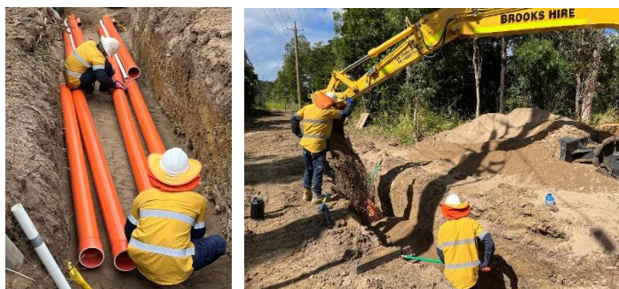
Fig 3 – Contractors joining and installing lengths of conduit at Flametree.
