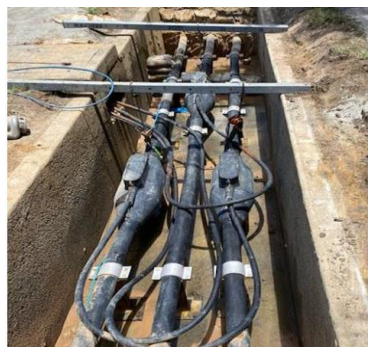
Fig 7 – Example of an underground cable joint bay.
