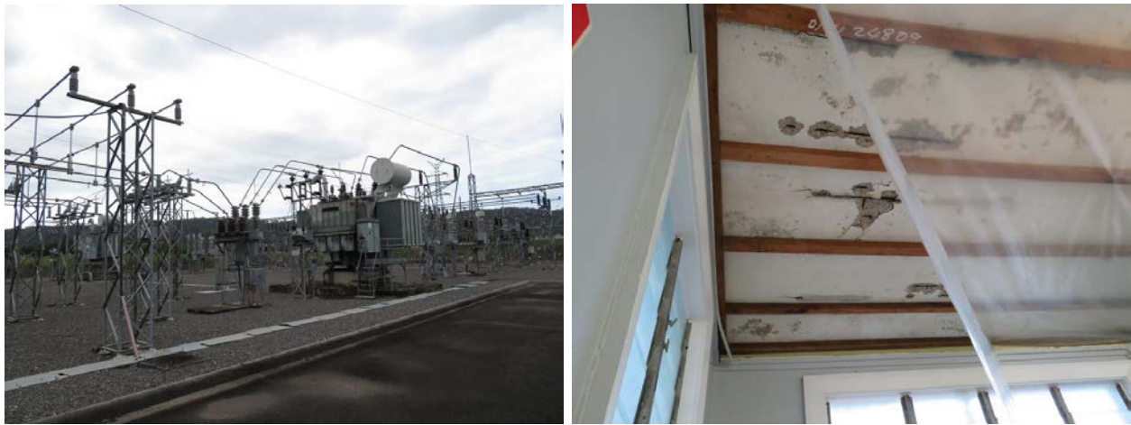
Figure 11 – Left: Mossman Substation yard showing aged plant. Right: Spalling of concrete ceiling exposing fully corroded reinforcement
