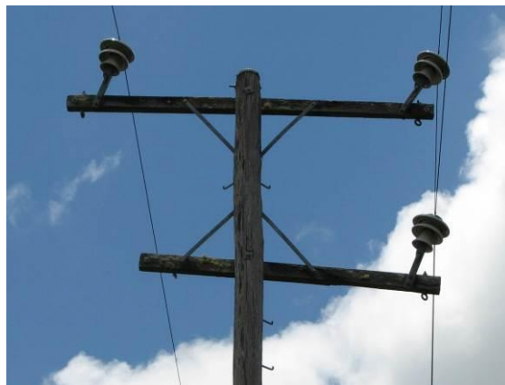
Figure 12 - 66kV delta pin construction
