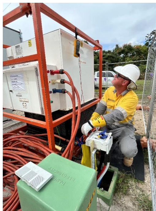
Fig 2 – testing the load bank before connecting it to the microgrid for testing and commissioning.
