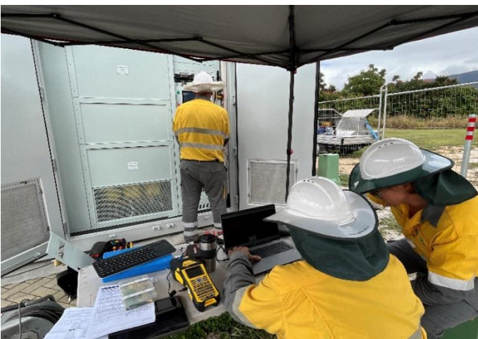
Fig 4 – The team fine-tunes the system and verifies the operating procedures during the microgrid testing and commissioning.
