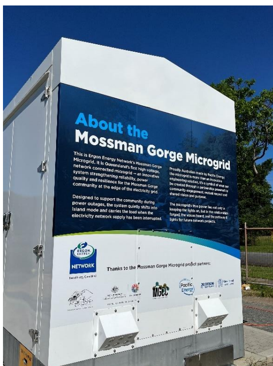
Fig 8 – Acknowledging our project partners.
