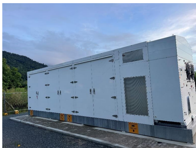
Fig 1 - The Mossman Gorge Microgrid's BESS unit before the wrap was applied.
