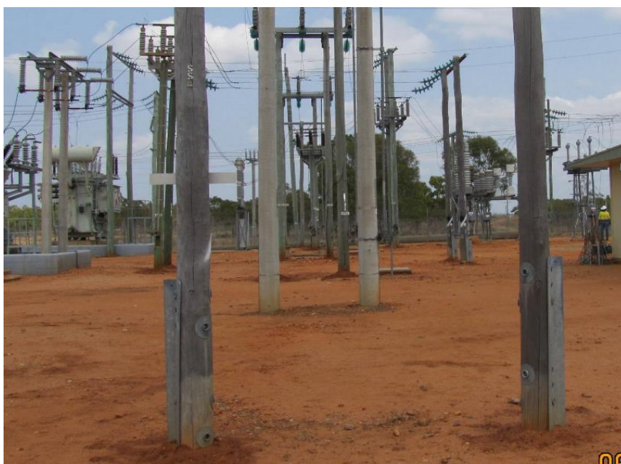
Figure 18 Photo showing pole nails on the 66kV supporting structures at CARI
