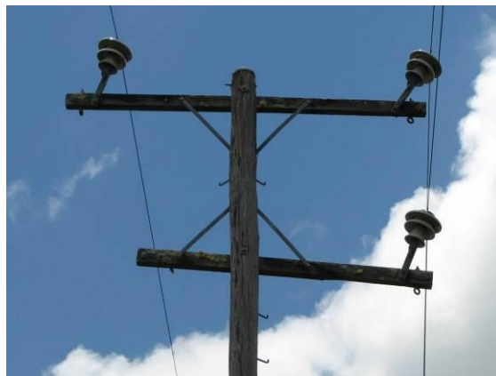
Figure 6 - 66 kV delta pin construction
