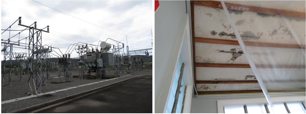
Figure 5 – Left: Mossman Substation yard showing aged plant. Right: Spalling of concrete ceiling exposing fully corroded reinforcement
