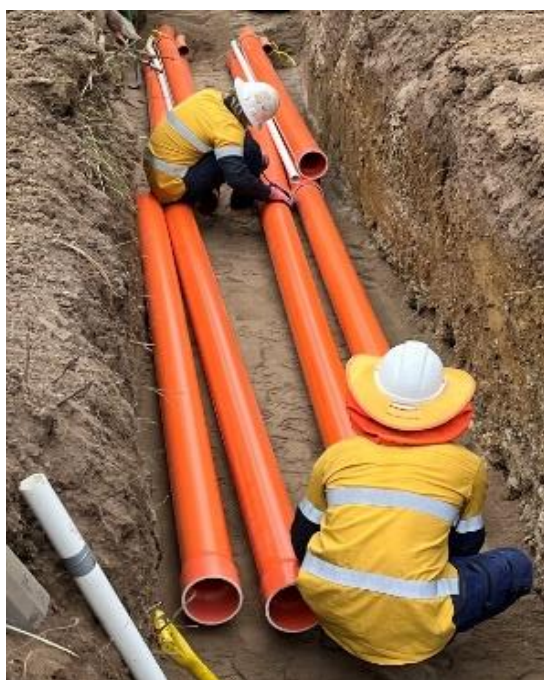
Fig 2 – Contractors installing lengths of conduit.
