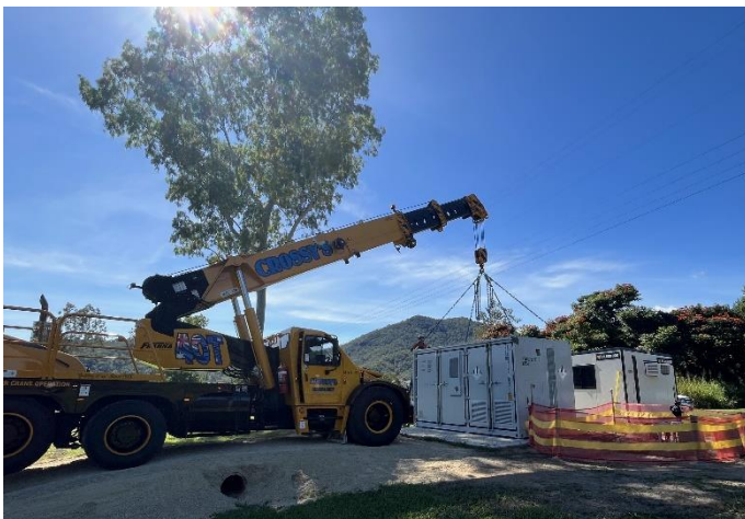
Fig 1 – The team from Crossy's Cranes lift the microgrid into place on site at Jumbun.
