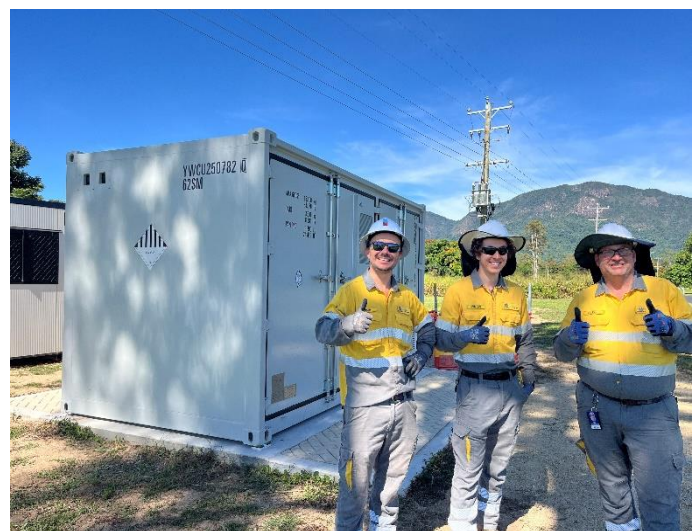
Fig 3 – A job well done! The Ergon team give the thumbs up for the safe delivery of the Jumbun microgrid.
