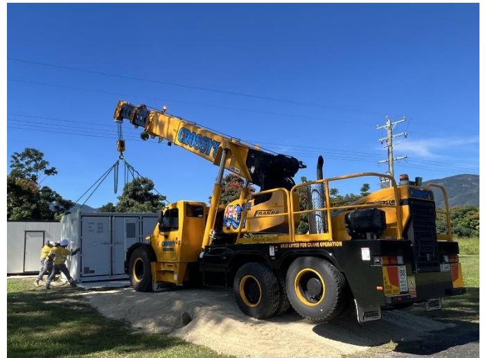
Fig 2 – It's a complex operation - the Ergon team work with the crane operators to manoeuvre the microgrid into place.
