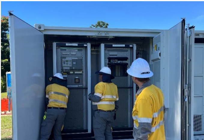
Fig 4 – The Ergon team unpack the microgrid and prepare to connect it to the surrounding electricity network.
