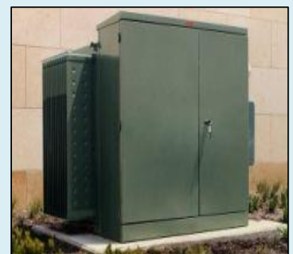
Figure 2: Above is an example of a pad mount transformer. This would not trigger referral to us.
