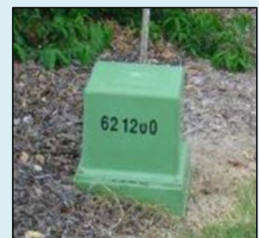
Figure 3: Above is an example of a service pillar. This would not trigger referral to us.
