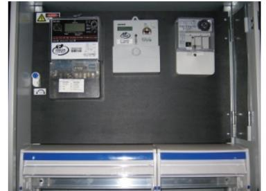
These have been designed for use in 'rock block' type construction sites and both enclosures are sized to fit the North Queensland concrete block format without the need for cutting.
