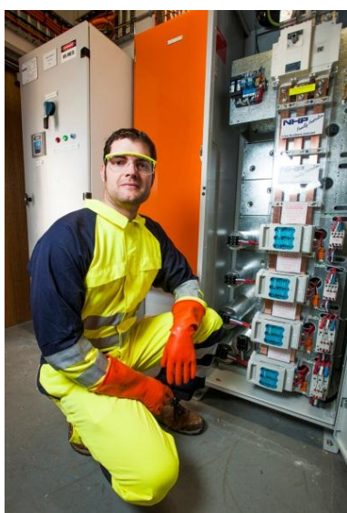
Above: James Glasby – Facilities Officer USQ Campus Services inspecting one of the eight capacitor banks installed
