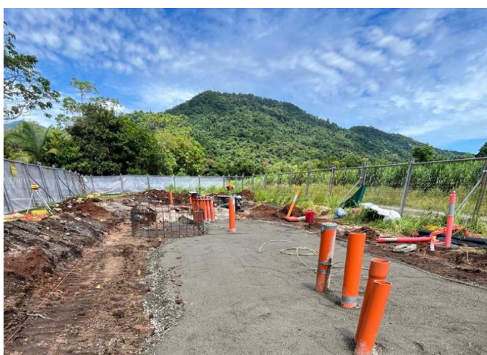
Fig 1 – On site, our civil works contractors are laying the conduits and foundations for the microgrid.
