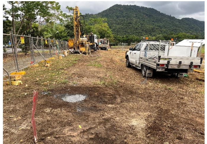
Fig 2 – Pot holes for the earth mat are complete and ready for the microgrid foundations to be constructed.
