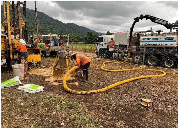
Fig 1 – Contractors use a vacuum truck to pothole the site.
