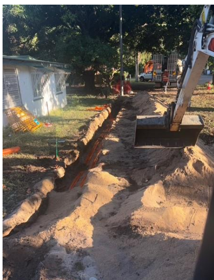
Fig 1 – Early civil works to install conduits were completed in June.
