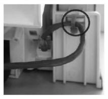
Bundle the Dred network cable at the wire-fixin hole of electric box with wire calmp . For 5.3kW is as below:
