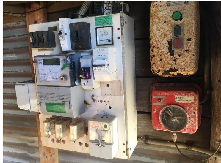
**Switchboard with load control signal receiver (bottom right) and Solar Analytics hardware (mid right) installed**
