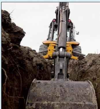
**Excavation works close to substation boundaries can cause earth movement around compound foundations, compromise protective earth grids and cause high voltage cable damage or exposure. These can all impact on the performance and safe operation of a substation and can be time consuming and costly to rectify.**
