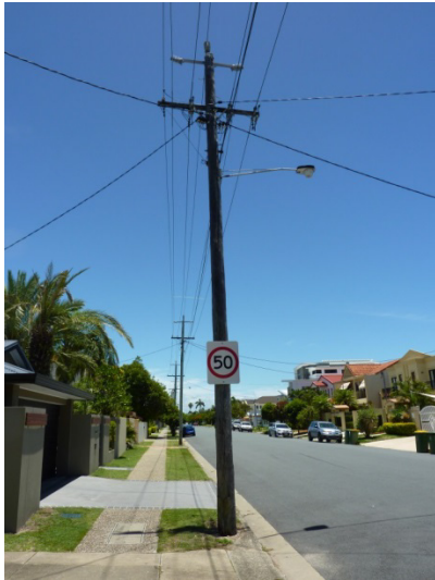
Figure 1: Representative Example - Authority Owned Signage Installation
