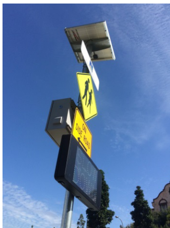
Figure 15: Representative Examples – Unacceptable Traffic Management Display Installations
