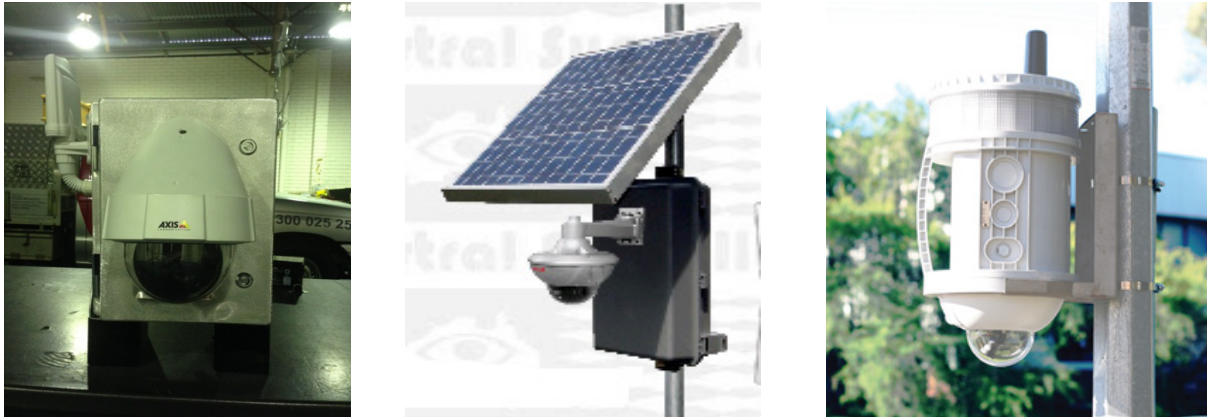
Figure 10: Representative Examples - Long Term Attachment Security Camera Installation
