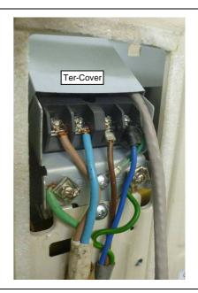
5 Fit demand signal wire to wire band (together with power cord wire).
