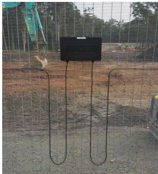
Figure 3 – PMII module mounted on fence
