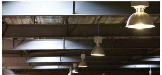
Above: The hi-bay lighting automatically switches off when there is adequate natural light penetration through the warehouse skylights.
