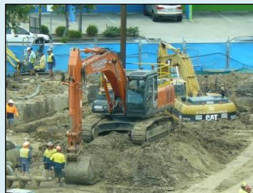
Filling works over underground cables can reduce the operating capacity and increase faults. This can also impact other assets within the network and subsequently incur additional maintenance and upgrade costs. Prior to the works starting, a cable rating assessment must be done to identify the operating limits of underground assets and ensures the network capital expenditure is spent appropriately.
