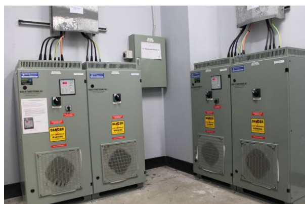
Power factor correction equipment at the main airport.
