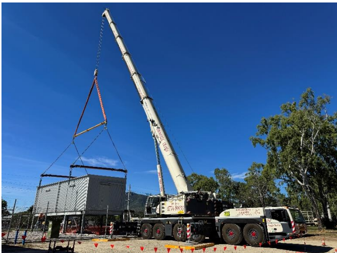
Fig 1 – A massive 300 tonne crane lifts the building into place.
