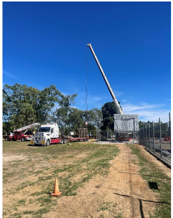
Fig 2 – Transport and crane operators and the Ergon team work together to manoeuvre the switching building into place.
