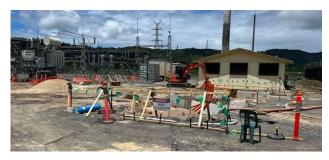
In preparation for the substation upgrade, works are also under way to establish a new underground communications network between key infrastructure, and to refurbish associated local 22kV powerlines.
