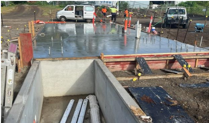
Fig 1 - Concrete foundation is poured and left to cure.
