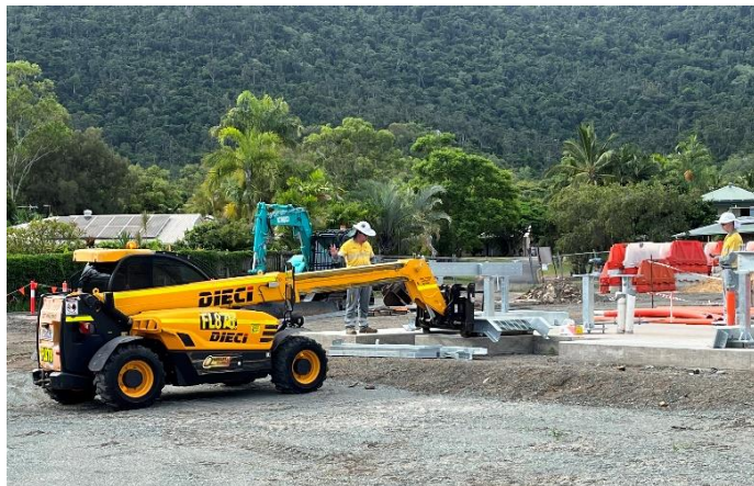
Fig 2 - Ergon crew prepares steelwork for the new control building.
