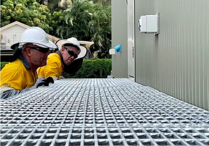
Fig 4 - specialised Ergon crew fit the steel verandas and staircases.
