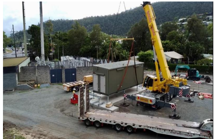
Fig 3 - Universal Cranes NQ lifts the building into place.
