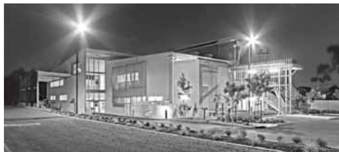
Ergon Energy's new $14 million training and development facility in Rockhampton was officially opened in May this year as a one-stop shop for the delivery of technical, field, safety, corporate and customer contact training.
