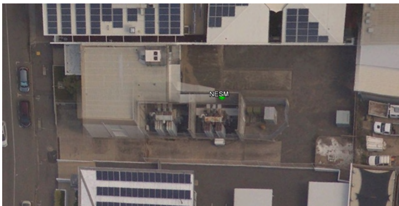
Figure 3: Neil Smith Substation (geographic view)
