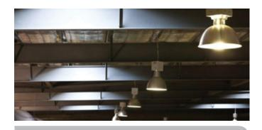
Above: The hi-bay lighting automatically switches off when there is adequate natural light penetration through the warehouse skylights.
