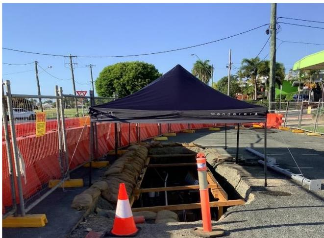
Fig 1 – 'Behind the curtain' - cable pit in Tennyson Street
