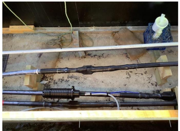
Fig 2 – Cables from the surrounding electricity network are connected to cables from the new substation.
