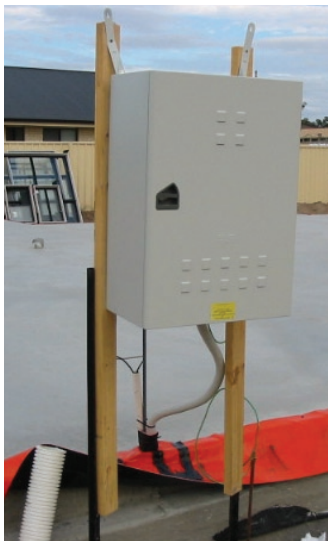
▲ Unacceptable mounting arrangement
