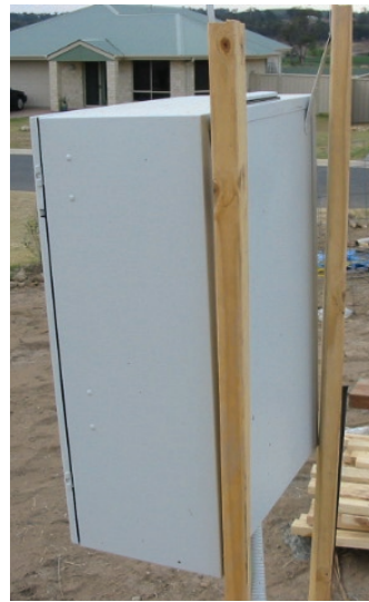
▲ Unacceptable mounting arrangement
