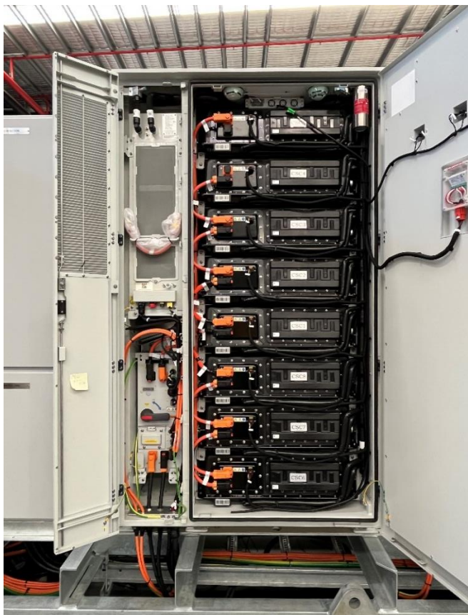
Fig 3 – Inside one of the BESS cabinets – several smaller batteries connected together
