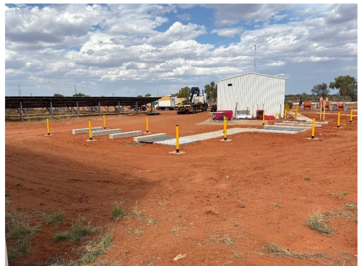
Fig 2 – Civil work for the BESS foundations and conduits is complete
