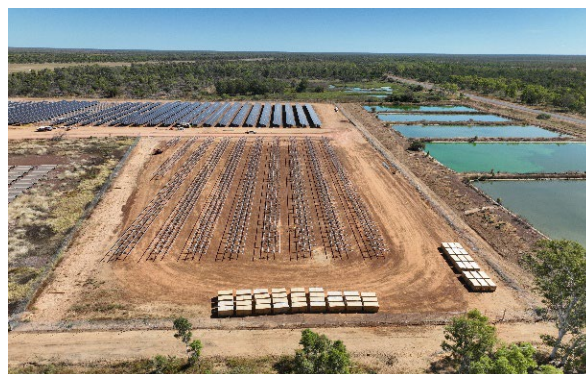
Aerial view of expansion works at Doomadgee of the solar and battery farm project
