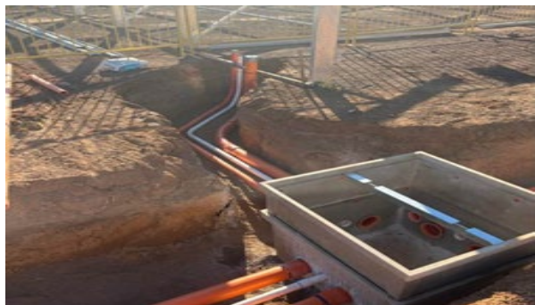
Installation of the underground cables that will connect the solar farm to the power station
