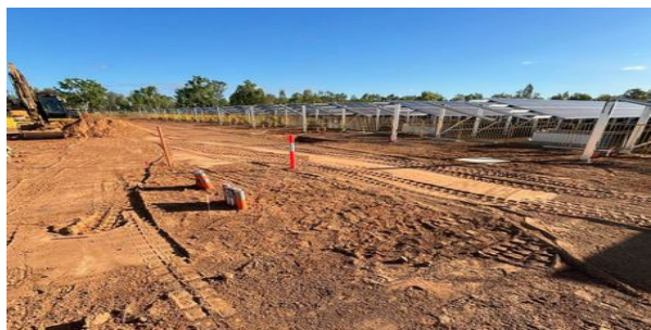
Installation of pilings
