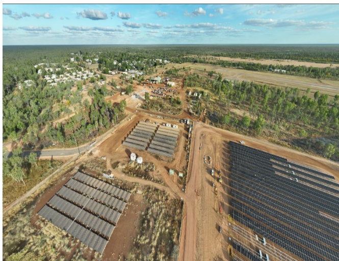
Birdseye view of expansion works at Doomadgee of the solar and battery farm project
