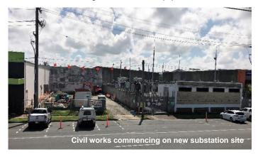
These preparatory civil earth works have included levelling out the parcel of land adjacent to the existing substation where the new substation equipment will be established and laying foundations for the electrical equipment. As well, blockwork for transformer bunding has been established, communications pits have been installed and temporary fencing has been installed for safety.
