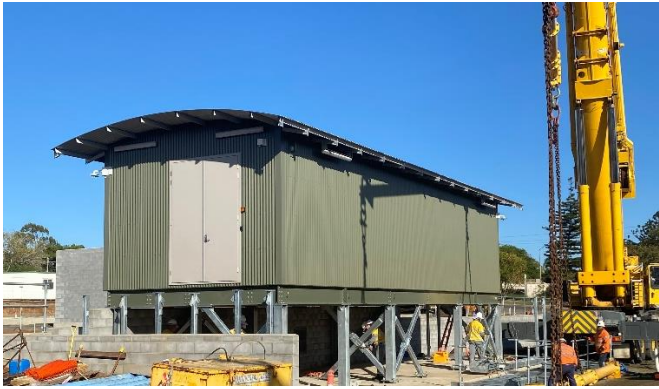
Fig 3 – The control building is secured onto the steel foundations.
