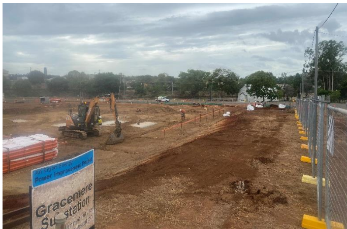
Fig 1 – Early civil works at the substation site commence.
