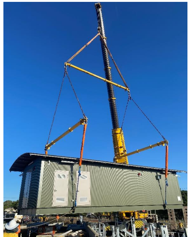
Fig 2 – New substation control building is manoeuvred into place.
