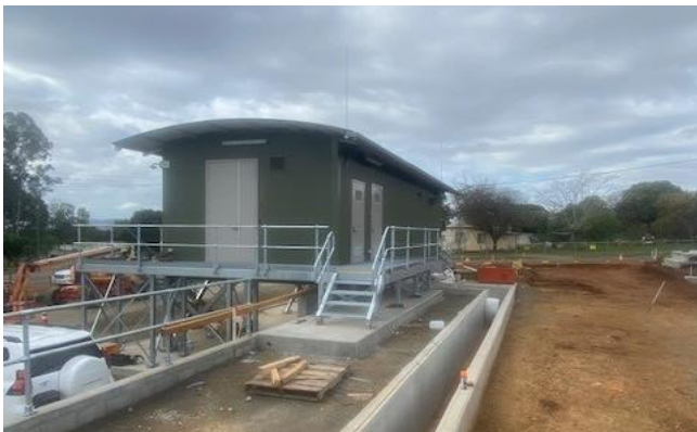
Fig 4 - The next stage of civil works commences in the substation.
