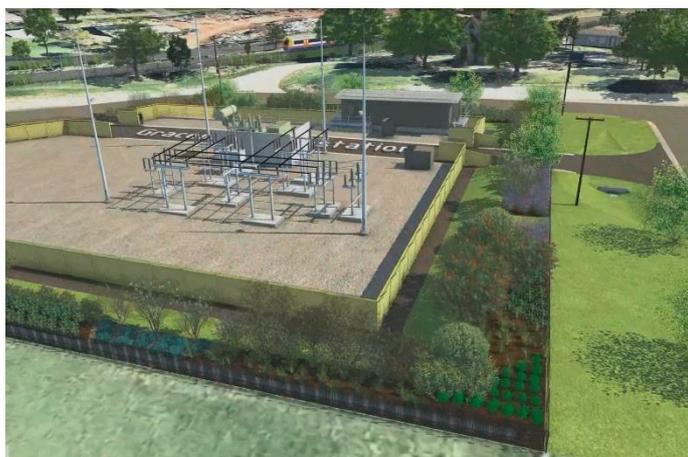
**Fig 3 – Example of dual fence construction around the new Gracemere substation**
