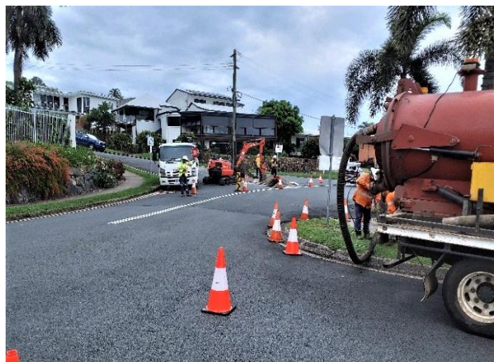
Fig 5 - Potholing to locate underground services down Mazlin Street into Broadwater Avenue before excavation commences.
