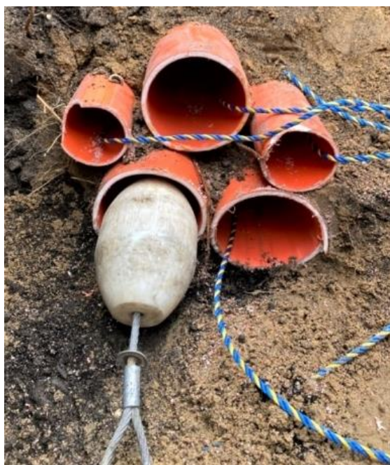
Fig 7 - A conduit mandrel used to clear debris from conduits.
