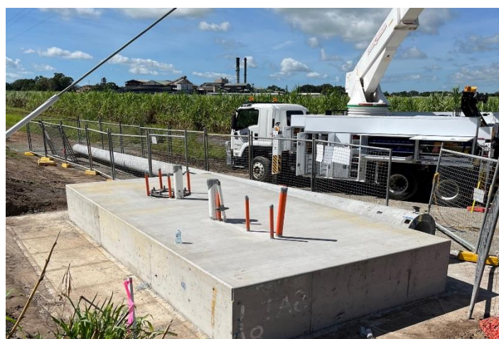
Fig 3- The foundations for the Proserpine communications tower are now complete.
