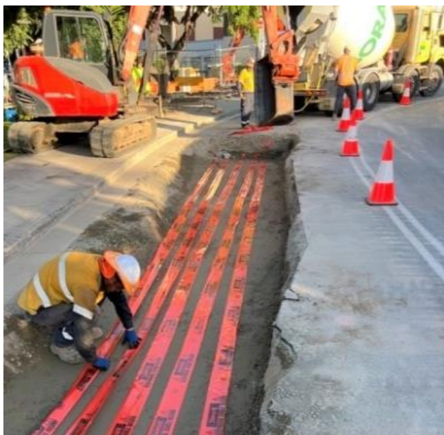
Fig 6 - Conduits are being installed along Broadwater Avenue for underground cables.
