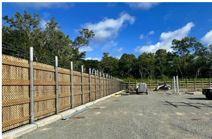
Fig 2 - New security fence being installed around substation.
