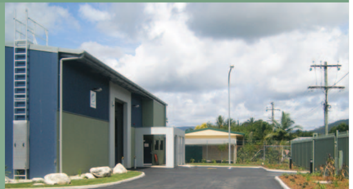
The Mossman depot in Far North Queensland was recognised with a Master Builders Award for Innovation in Environmental Management – captured water is used for toilets, water run-off is filtered, energy efficient lighting is used throughout and the building is fully insulated.
