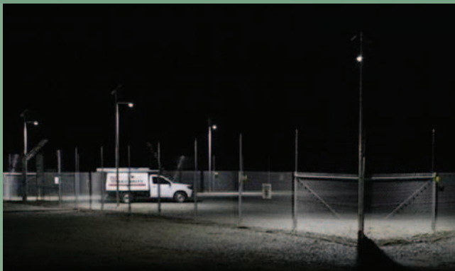
New solar-powered LED lighting has recently been installed at Ergon Energy's Pandoin Substation storage yard. The energy-saving LED lighting is rated for 100,000 hours – or 20 years – before a bulb change is required.
